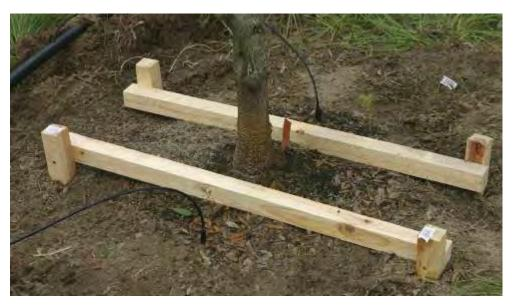
FIG. 19 BIODEGRADABLE ROOT ANCHOR USING UNTREATED TIMBER
