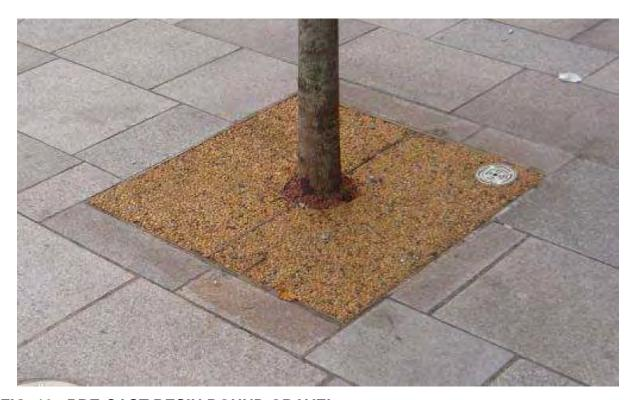
FIG. 13a PRE-CAST RESIN BOUND GRAVEL
